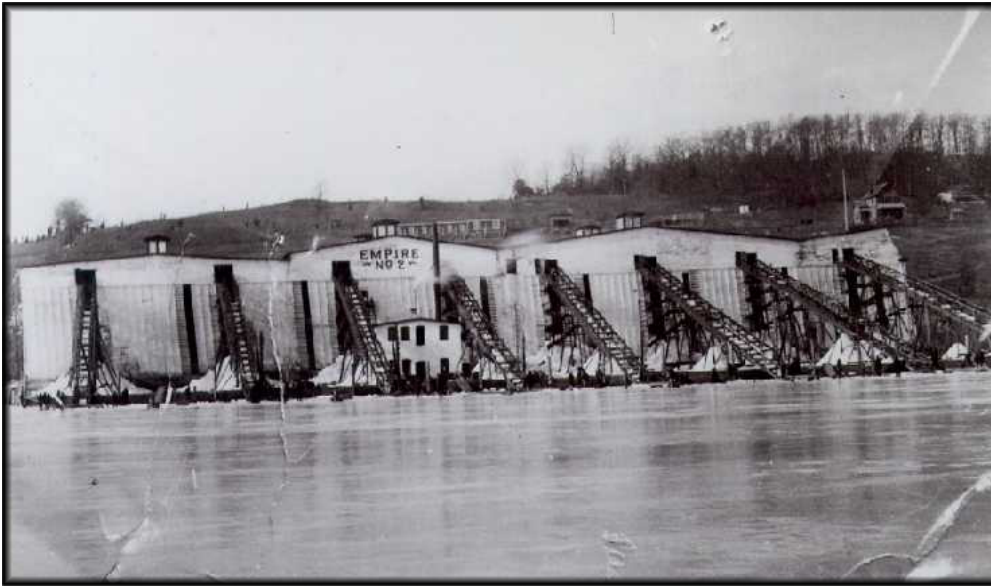
Figure 21. Substantial variation existed among Hudson River ice houses in the configuration of elevators used to load ice. Here, in an undated photograph of the Empire Number 2 Ice House at Catskill, N.Y., a separate elevator is located in front of each door. (Courtesy of the Vedder Memorial Library, Greene County Historical Society.)
